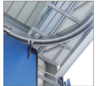
Curved top track to suit building profile allows door to return back into the building and be stored neatly minimising space requirement
