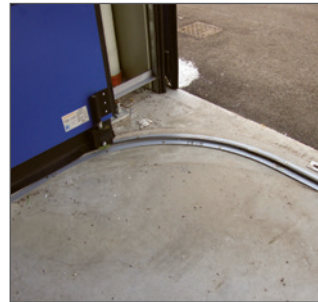
Bottom track manufactured and cost in to suit top track position
