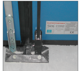
Integrated shoot bolt and wicket door keep
